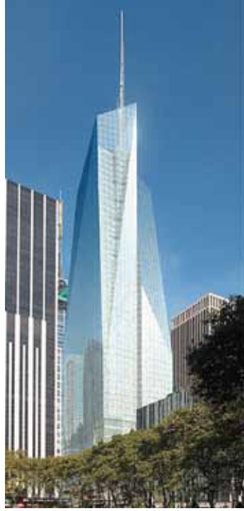
One Bryant Park, New York LEED Platinum Sertifika
